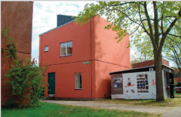
At Hylde-spjældet the first zero energy housing renovation in Denmark was realised in 2009 introducing prefabricated construction elements from Rockwool and the Solar Prism installation element.
