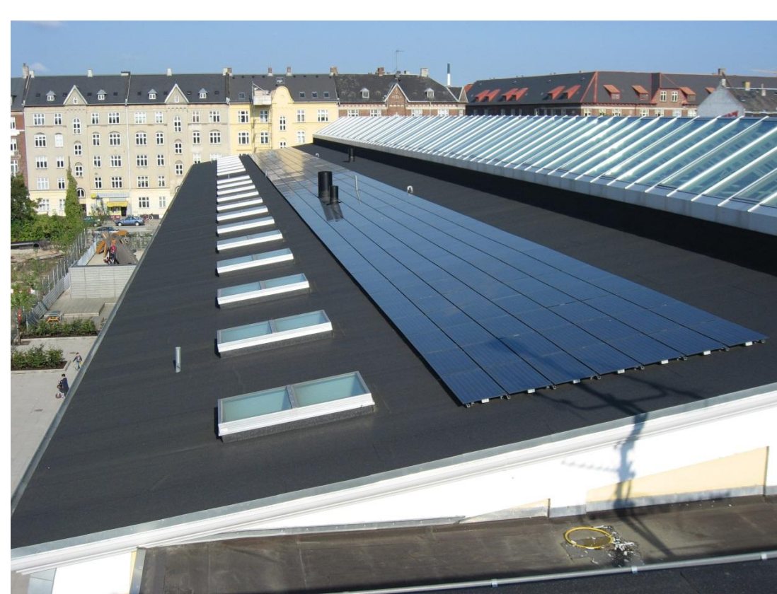
Valby School in Copenhagen with BIPV ( Building Integrated Photo Voltaic )
