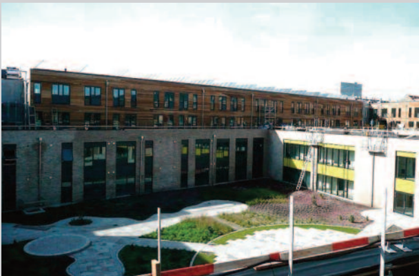
Langgadehus housing area in Valby with 200m 2 solar thermal collectors
