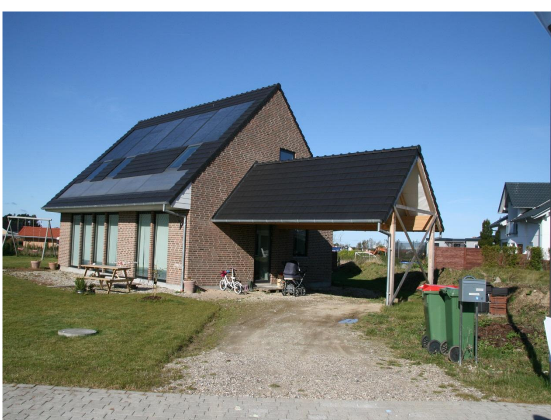
Development of low energy buildings in Stenløse, DK, as part of EU Concerto Project Class1.
