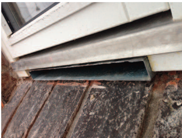
The new windows for the test apartment was supplied by the Danish EVD company with built in fresh air intake and used air exhaust integrated in the bottom of the window equal to \varnothing 140 mm.
